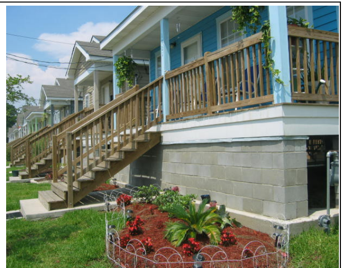
Completed Habitat for Humanity homes. Part of the Musicians' Village in the Upper Ninth Ward.
